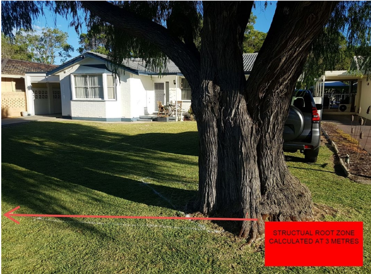
Photo 1 (provided by applicant)
